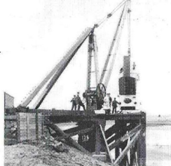
A vertical boiler is prepared for loading on-board ship.
