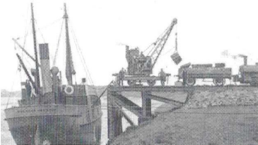
A Cochran powered crane unloading press-blocks at Newbie Pier 1899 of the twentieth century. The present 52 acre site in Dumfriesshire, Scotland, was selected in 1897 as it had suitable slipways for the small ships the company built.
