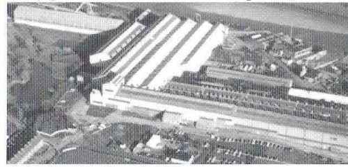
Aerial view of Newbie works 1977
